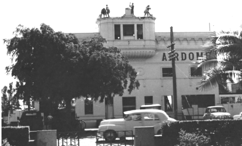
Demolition under way at the Olympia Airzone
